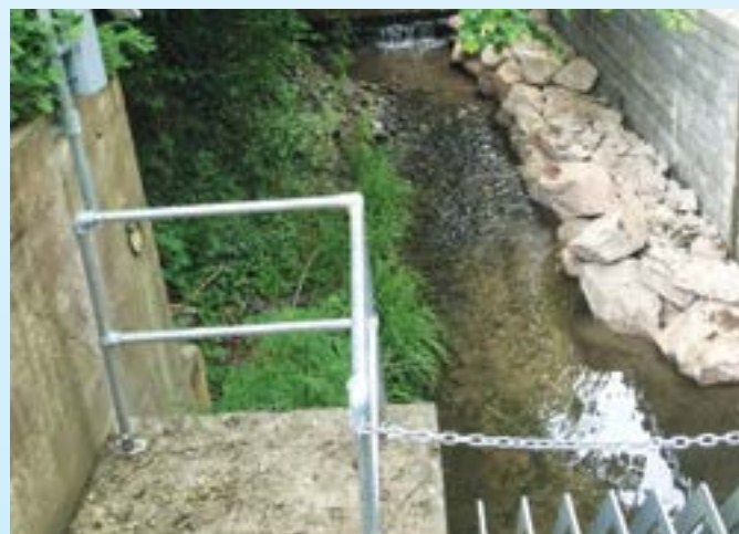
Plate 3 – The new Brislington Brook retaining wall reducing fluvial flood risk
